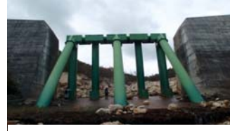
Figure 4(a). The open check dam in the Hachimandani River.
